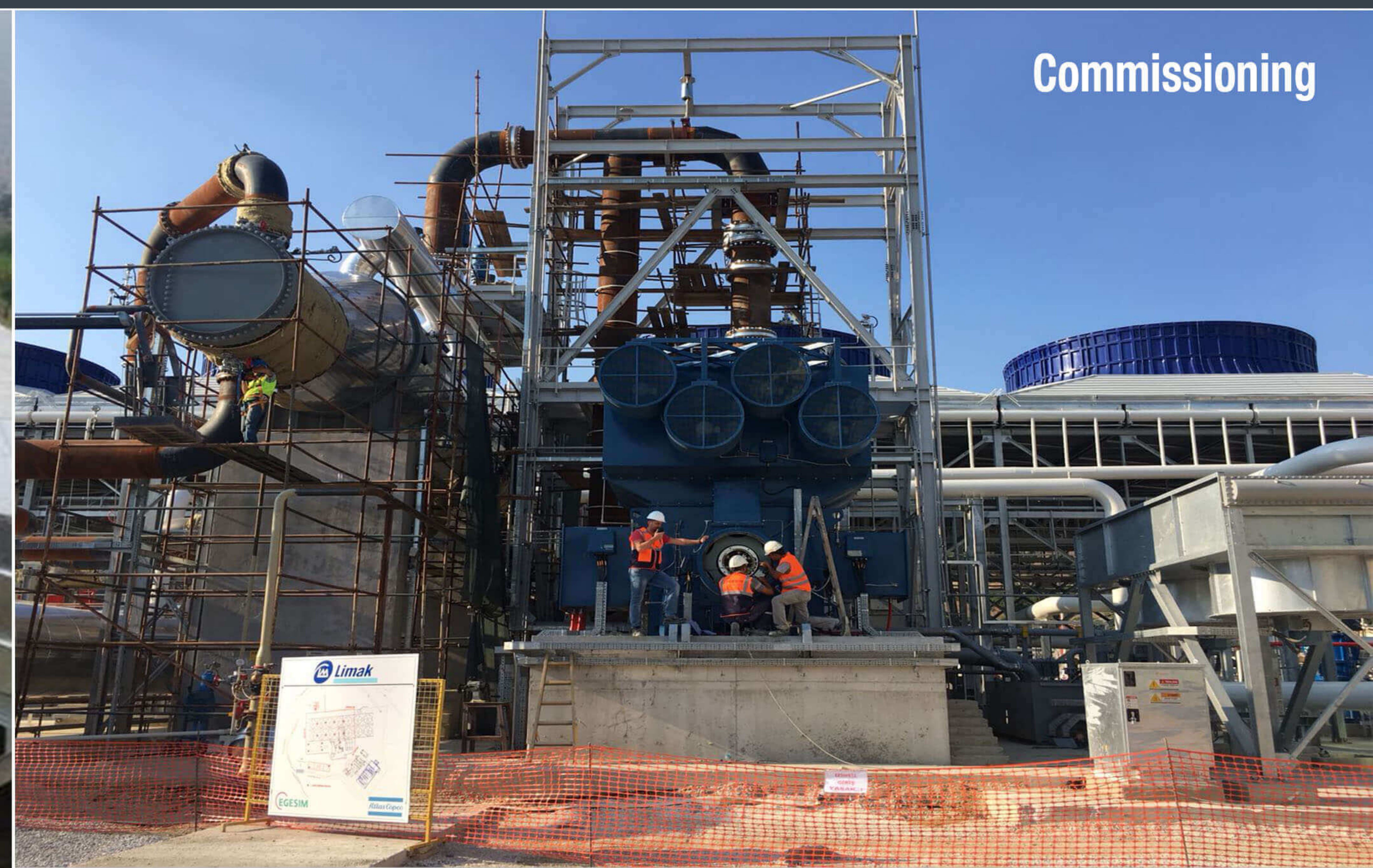
Installation at site
