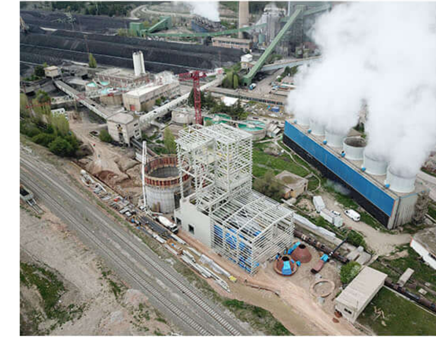
Thermal Power Plants
